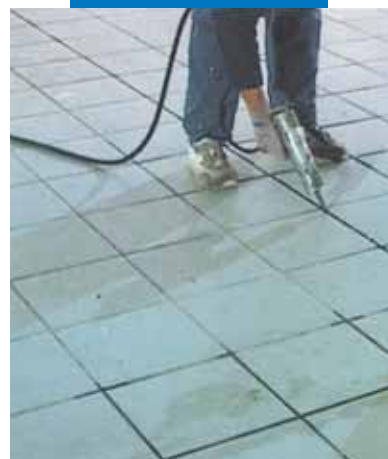
Sealing ceramic tile floor with Mapesil AC
